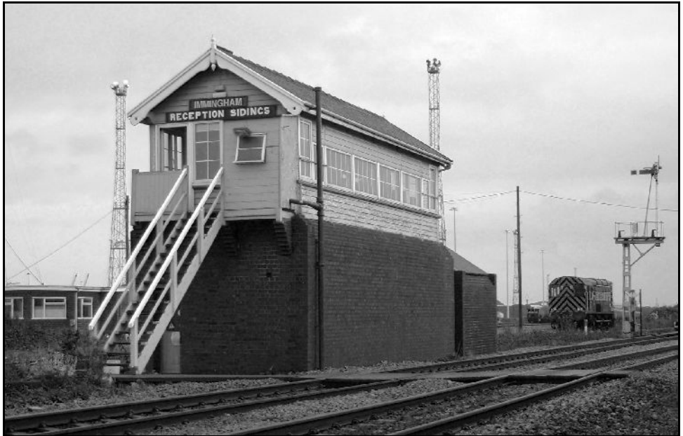
Immingham Reception Sidings signal box.
