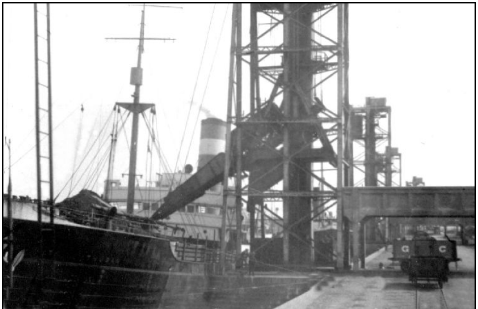
Coaling at No.2 hoist. A wagon is being end-tipped on the hoist while the previous wagon stands on the lower level empty wagon shunt neck. There also appears to be a low-sided wagon on the dockside photo: Immingham Museum
